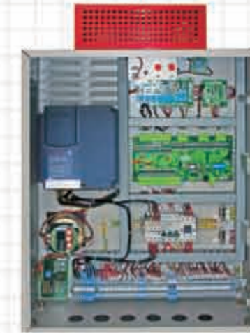
INTELLIGENT 32 BIT MICRO CONTROLLER & IMPORTED AC VVVF OPEN LOOP / CLOSED LOOP DIGITAL FEEDBACK DRIVE BASED CONTROL SUITABLE FOR MACHINE ROOM APPLICATION
